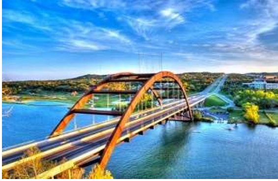
The Pennybacker Bridge in Austin is a through-arch bridge across Lake Austin which connects the northern and southern sections of the Loop 360 highway, also known as the "Capital of Texas Highway."
